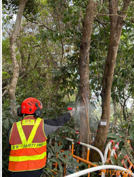
18: Spraying of termiticide
