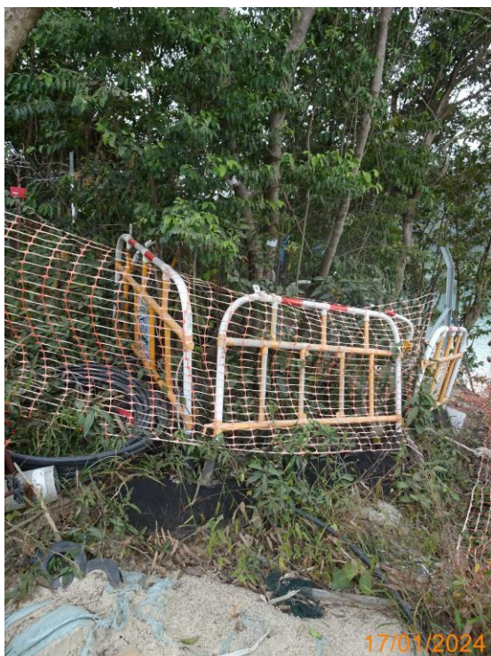
19: Slit rock and protection zone
