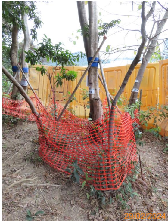
20: Temporary protective fencing for U041, U042 and U043
