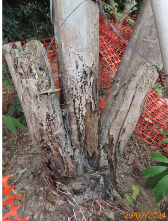
10: U041_Wood damage at trunk union
