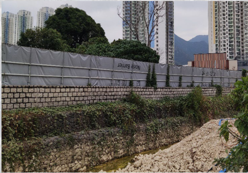
Deployment of noise barrier
