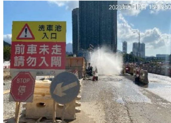
Wheel washing bay with high pressure jet
